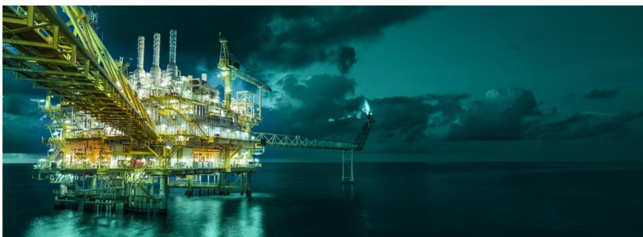
E-house modules for emergency power system for Offshore installations.
