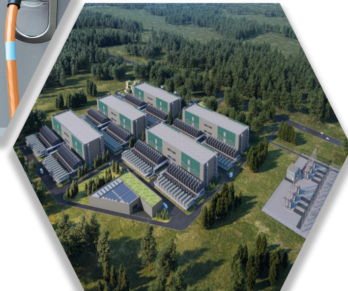
Datacenter Emergency Power
